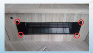
2. Use sharp-nosed pliers and other tools to remove the wire that secures the ends of the heating tube.
