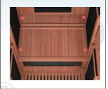
11. install the backrest and fix it with ST4\*50MM\*2pcs screws.
