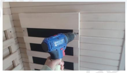
2. Carefully remove the heater, find the connector between the heater and the sauna wall, disconnect the connector between the heater and the sauna wall, and use a screw-driver to remove the screws that hold the heater to the wooden fence.
