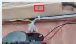
After connecting the power cable, the position of the frame is fixed with ST 4*40mm*4pcs screws.
