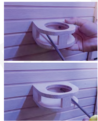
15. Install the tea cup holder and fix it with ST3.5*25MM*2pcs screws.
