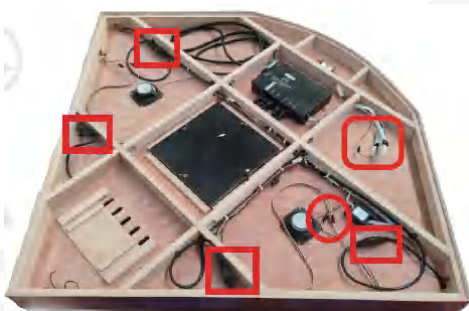
16. Power cord connection on top of sauna.
